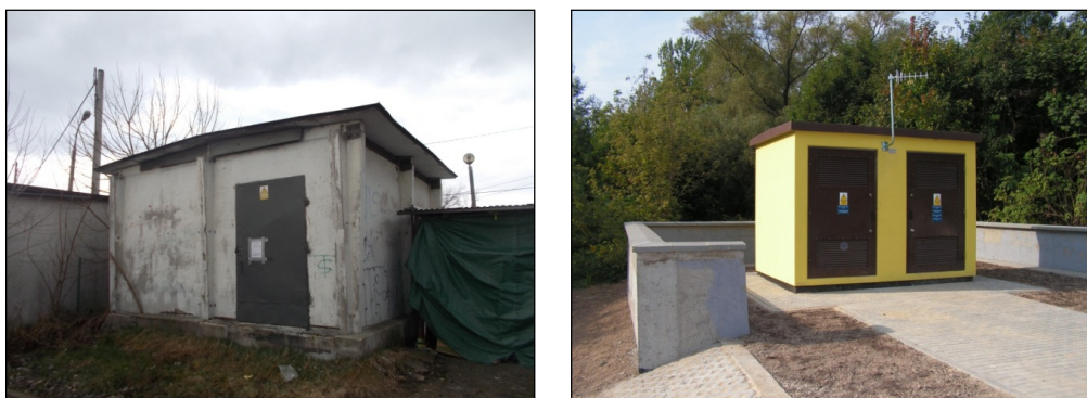
Fig. 1. Examples of transformer stations in the area of Krakow (source: own materials)
