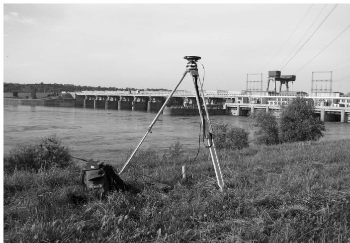
Fig. 1. Włocławek power plant
