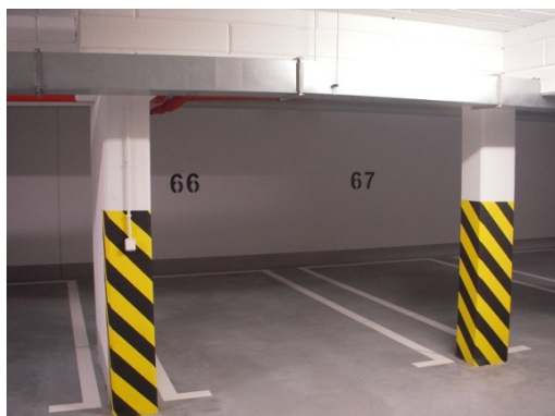
Fig. 1. Parking space in the underground multiposition garage (source: author's own archive)
