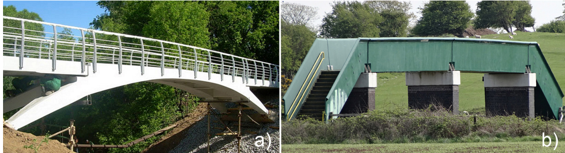
Fig. 5. a) Arch footbridge in Moscow, Russia (Source: www.apatech.ru), b) Bradkirk Bridge in Kirkham, UK (Source: own image)
