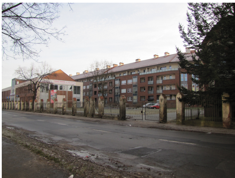
Fig. 3. Housing estate “Wawel Estate” Photo by Rzasa K. 12.2016
