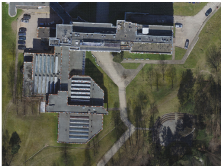
Fig. 7. Rooftop and objects in detail. Orthophotographic view
