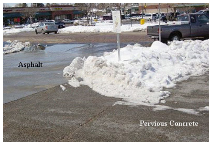
Fig. 6. Comparison of pervious and impervious surface during winter season
